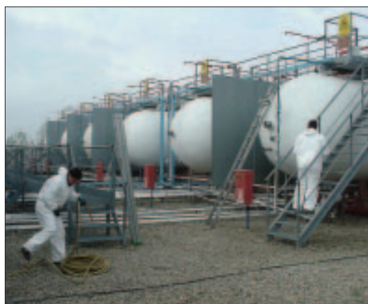
Bonifica serbatoi GPL
